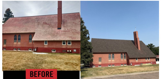
Pictures from KQC Roofing
